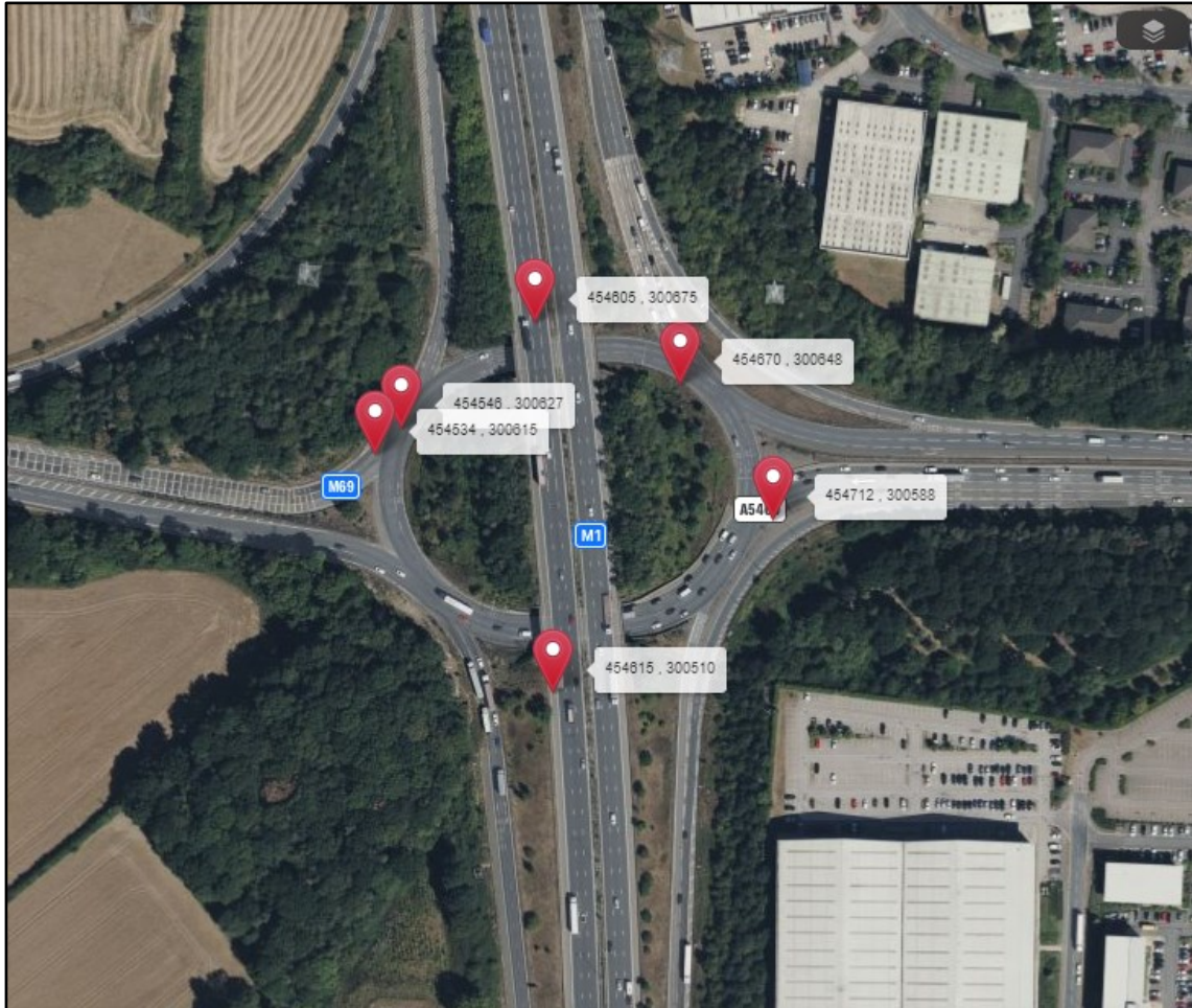
Figure 3.7: M1 Junction 21 Roundabout
