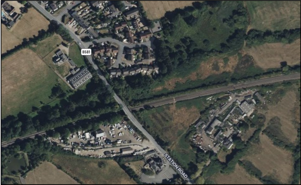
Figure 2.12. Station Road Railway Overbridge Elmesthorpe
